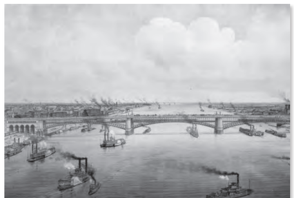
Figure 2.6 St. Louis Eads Bridge
